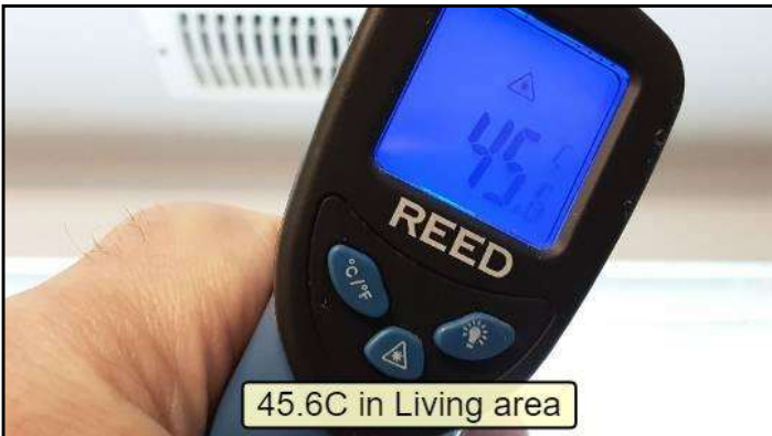
14. Furnace air flow and temperature taken at the
